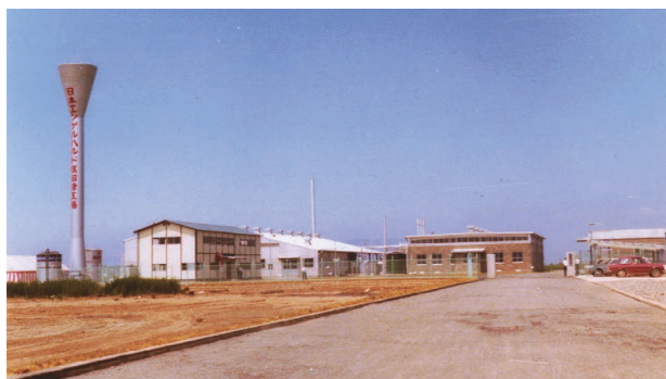
Numazu Factory at the start of operations
