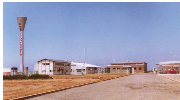
Numazu Factory at the start of operations
